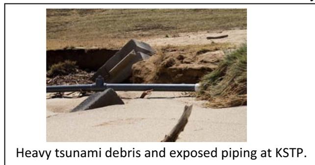
Heavy tsunami debris and exposed piping at KSTP.
